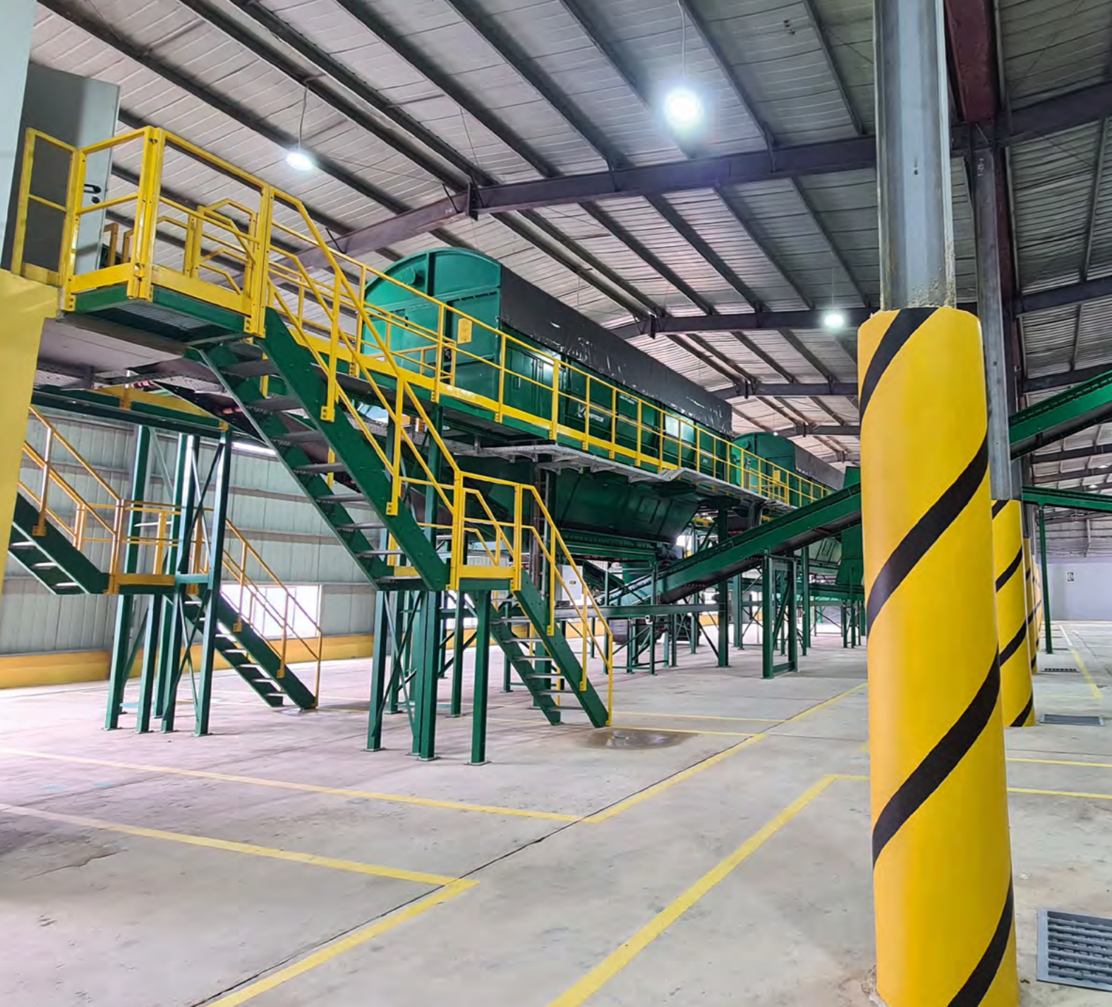
Integrated Recycling And Compost Plant (IRECOP) – Location: Accra, GHANA Start of operation: 2019 Capacity: 200 tons per day
